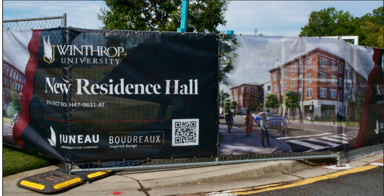
Sign at the construction site of Winthrop's new residence hall Photo by Zoey Molina
