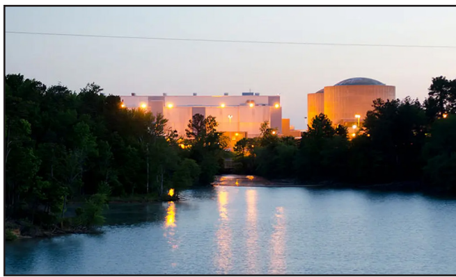
Photo via Carolina Country Outside view of the Catawba Nuclear Plant
