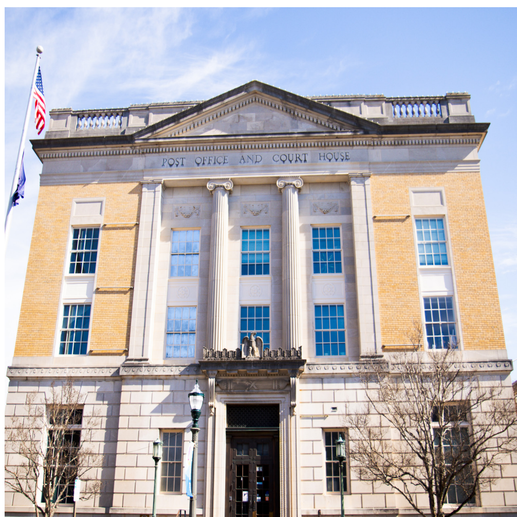
Outside view of the Tom S. Gettys Center, with the "Post Office and Court House" sign in view photo by Jackson Stanton
