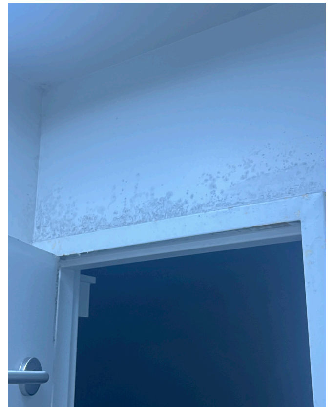
Mold above a door in a student's dorm room photo by Kaydence Hill
