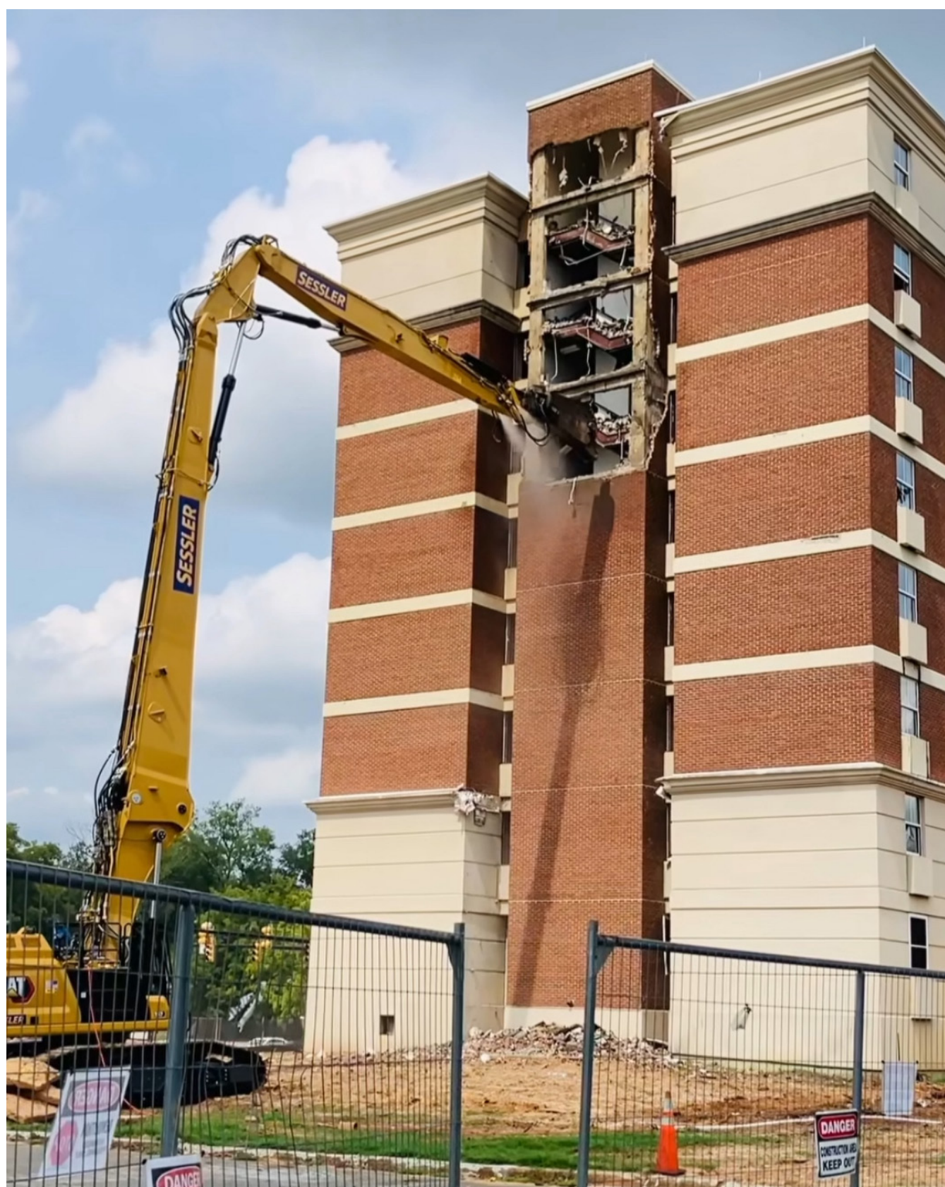
An excavator tearing down Wofford Hall.
