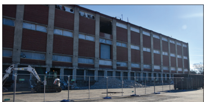
According to Jon Little of Choate Construction, the front of the building will go from fully brick to being covered with glass windows.
