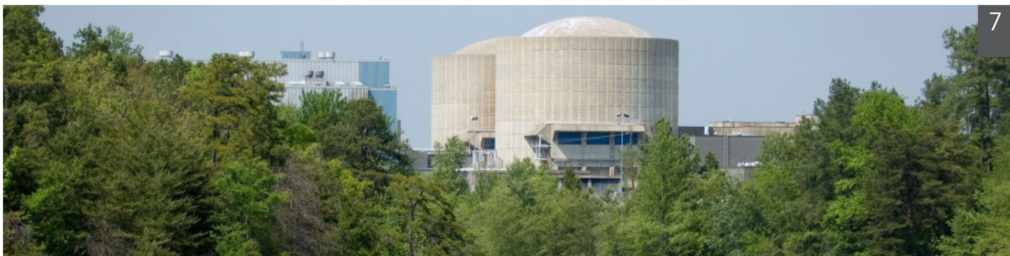
The twin pressurized water reactors of Catawba Nuclear Station on Lake Wylie
